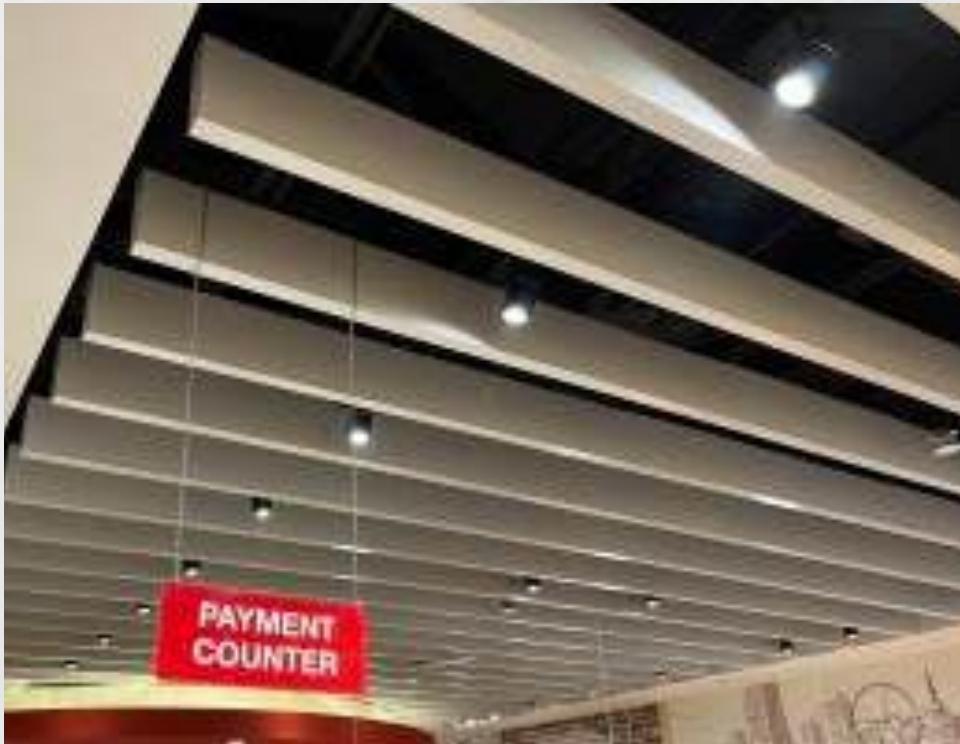
F&B RESTAURANT CEILING
