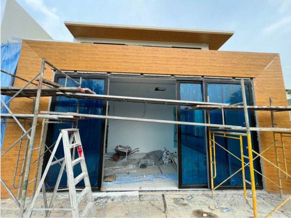
CAR PORCH, ROOF & CLADDING
